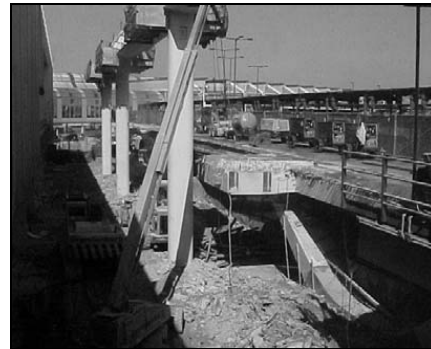
O'Hare FACE Project: Terminals 2 & 3 Chicago, Illinois
