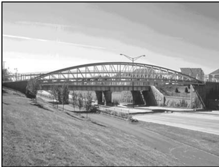
BNSF Railroad and Gilman Trail Bridges over Orchard Road, Aurora, Illinois
