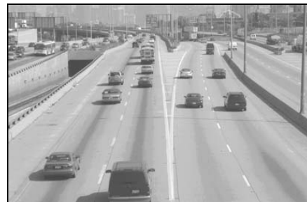
Dan Ryan Expressway Reconstruction Chicago, Illinois
